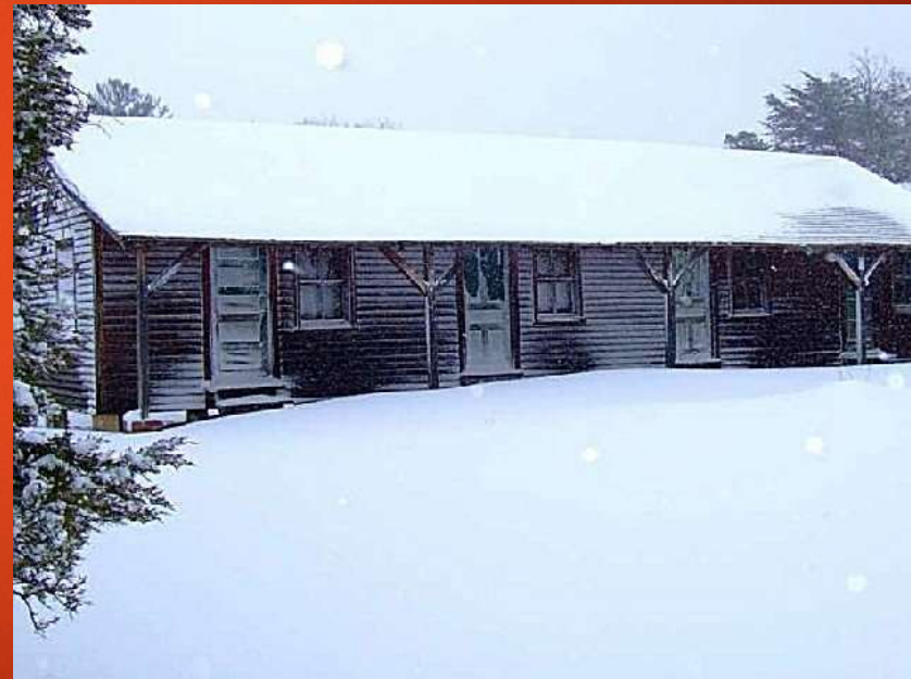
BUNK HOUSE FOR SINGLE MEN AT DOUBLE TROUBLE
